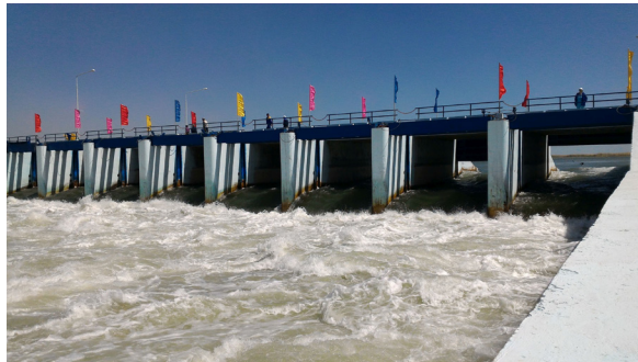
Fig. 4 The Kokaral Dam feeding the Central Aral.
