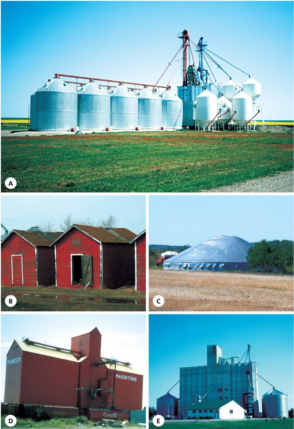
Fig. 1. A, Corrugated metal bins are one of the most common farm grain storage units. Hopper bins (white) allow for easy unloading. B, Wooden bins are still used occasionally. C, There are many types of temporary storage units. D, Wooden elevators covered with metal sheathing were built from 1920 to 1960. E, High-throughput concrete elevators or inland terminals are quickly replacing the smaller wooden elevators.
