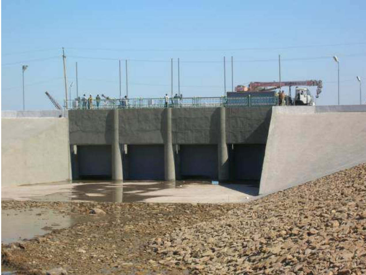
Special water way and water discharge gates just after construction in September 2005. Photo by P. Micklin
