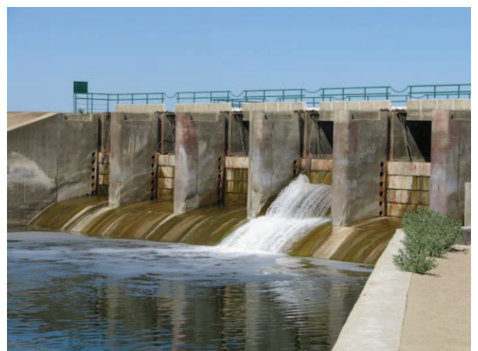
Fig 11: Two views of the spillway of the Kokaral dam ©I. Aladin
